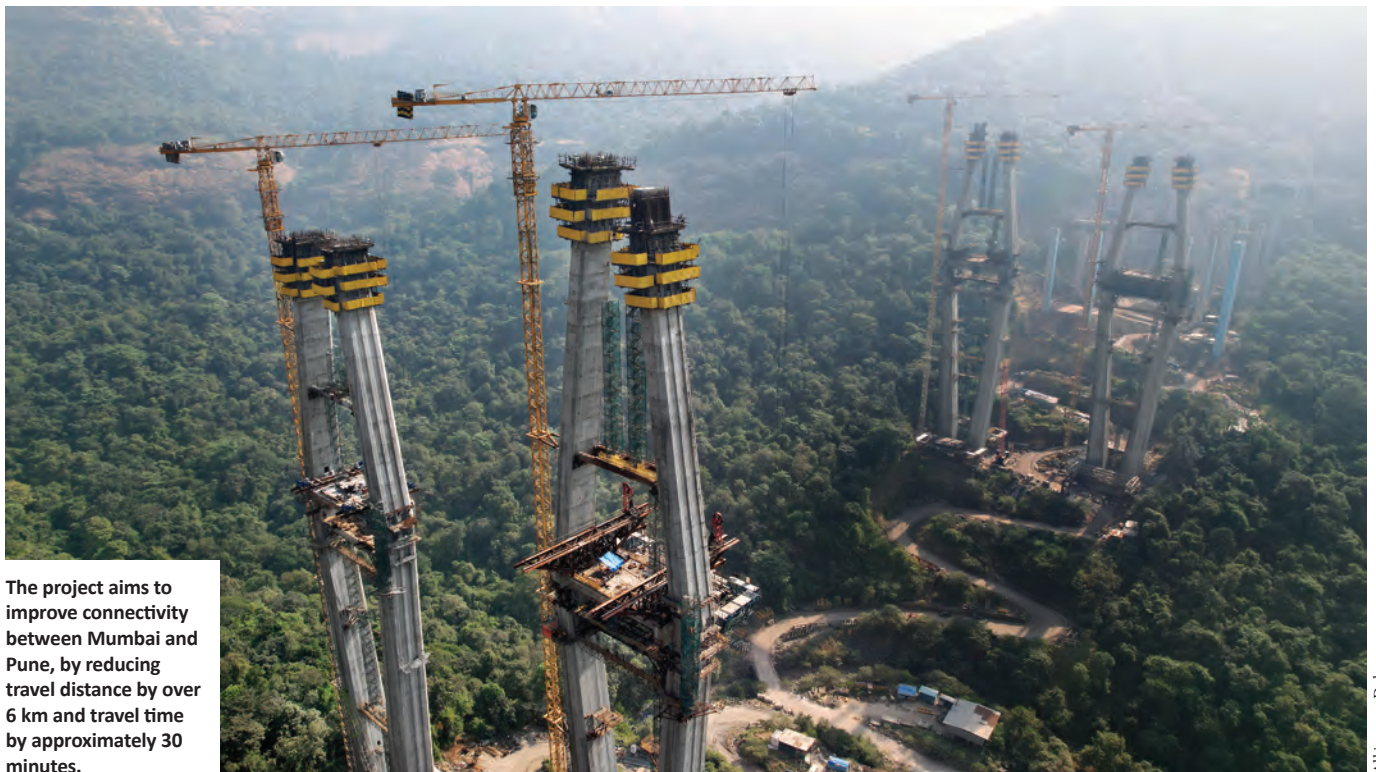
The 650-m-long cable-stayed bridge features four diamond-shaped pylons, each 181.77 m high – making it one of the tallest in India.
