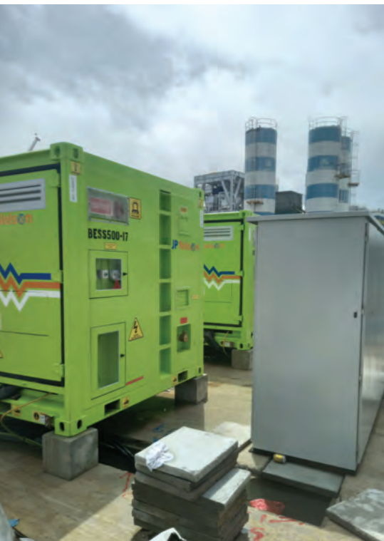
ABOVE AND LEFT: JP Nelson has deployed several units of its battery energy storage system (BESS) on construction sites in Singapore. This system is environment-friendly, reducing reliance on fossil fuels and greenhouse gas emissions. It also enhances the reliability of renewable energy sources.
